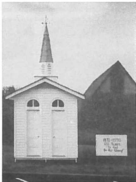
Replica of 1870 Building
