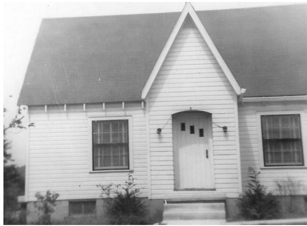
Above: Oneida church of Christ Parsonage built 1947 Below: Same house in another location 2008
