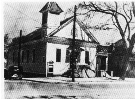
1 st West End Ave. Bldg.
