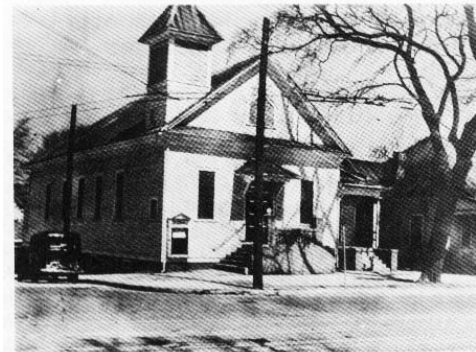
1 st West End Ave. Bldg.
