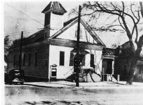
1 st West End Ave. Bldg.
